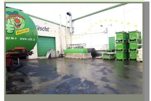
Washing area with oil and grease separator
